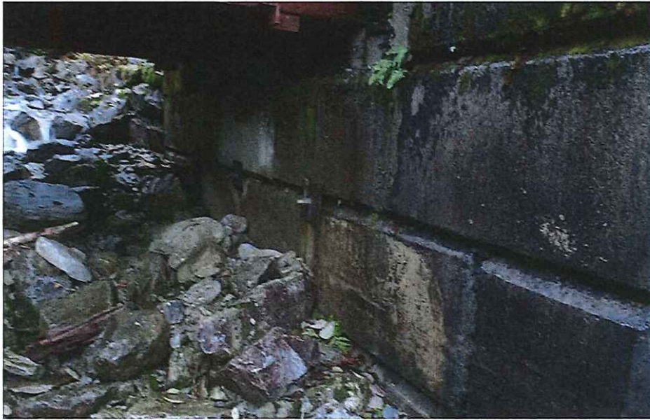
CK2327 Left Abutment
