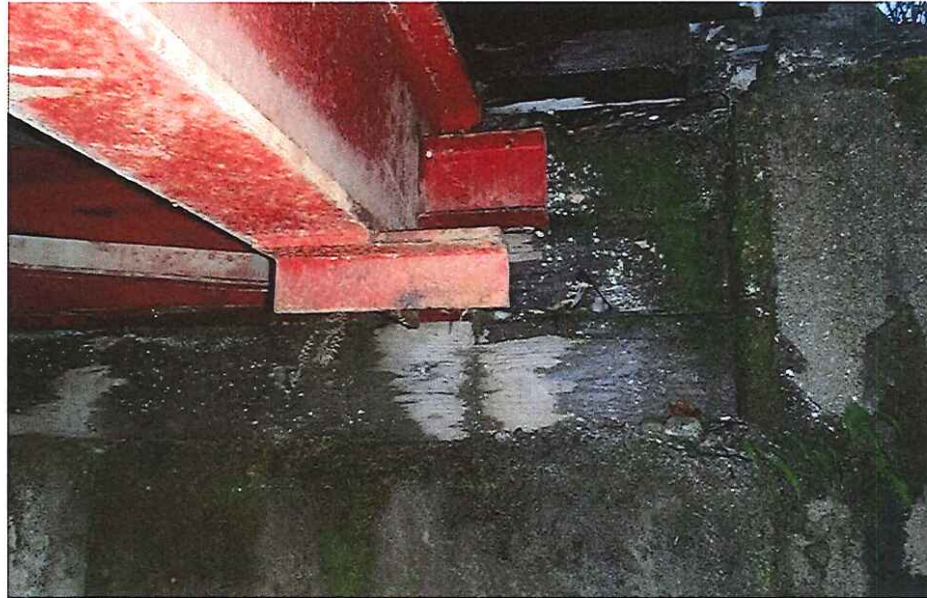
CK2327 Left Abutment bearing
