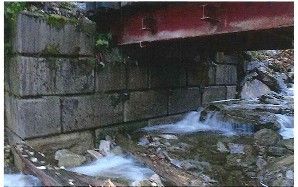
CK2327 Right Abutment
